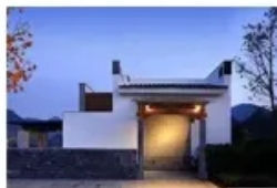
Household Energy Storage
