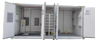
1075KW HH ESS
