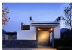
Household Energy Storage
